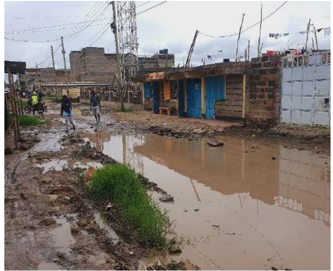
Urban flooding caused by lack of drainage channel in Mlolongo Central area
