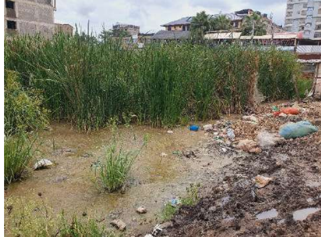
Waste on the drainage channels
