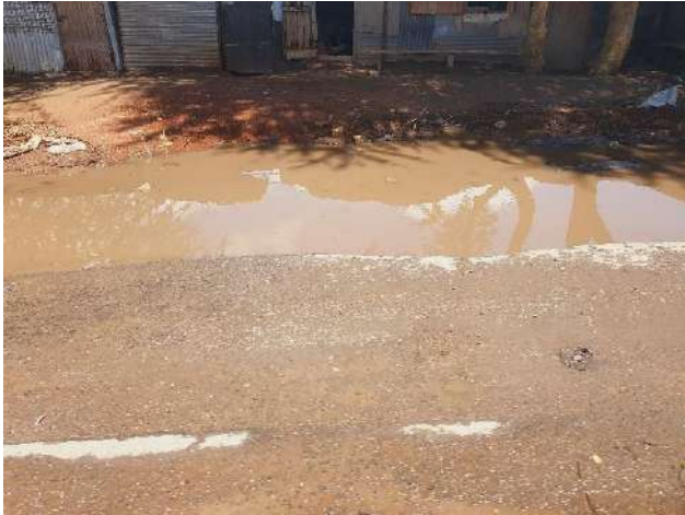
Urban flooding due to lack of proper drainage channel along the road in Athi River central area
