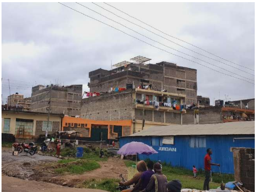
Flats in mlolongo urban area
